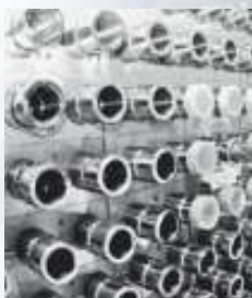
Calandria Channels with END FITTINGS of Nuclear Power Reactor
